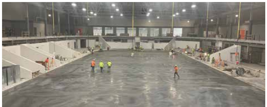
Vee-Jay Cement Contracting created three ice rinks for the same customer
