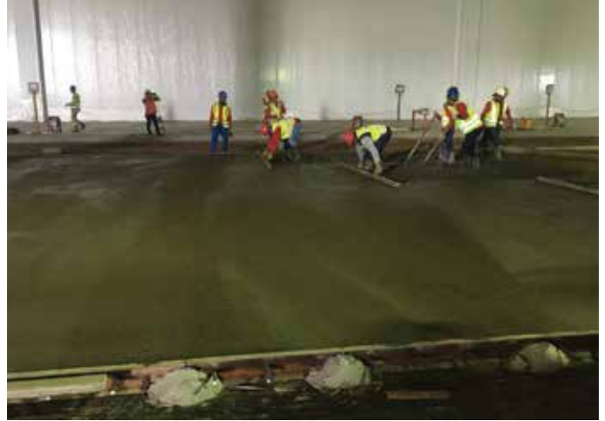
Crew from Europiso Comercio de Pisos Industriais hand-striking off a floor
