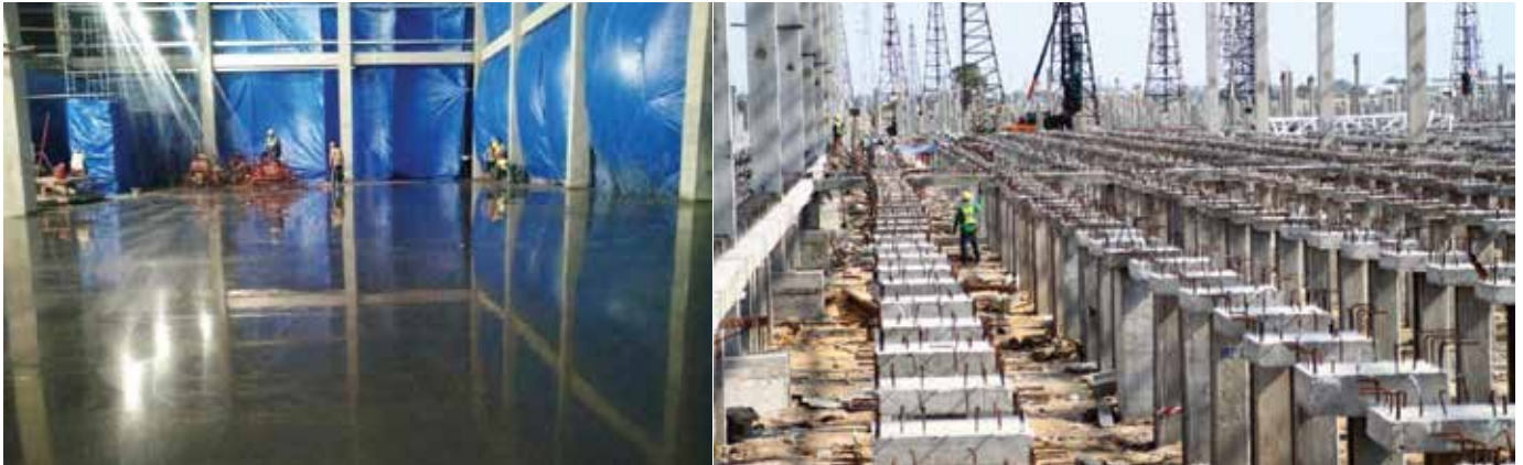
B.S.Y. Construction Co. constructed an elevated floor supported on piles
